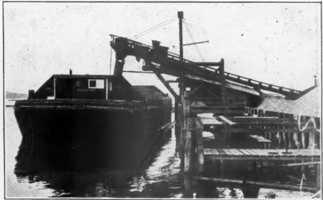
Loading a Barge
